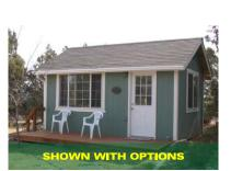
6/12 PITCH ROOF, 2"X6" JOIST, 3/4" PLYWOOD SUB FLOOR,
